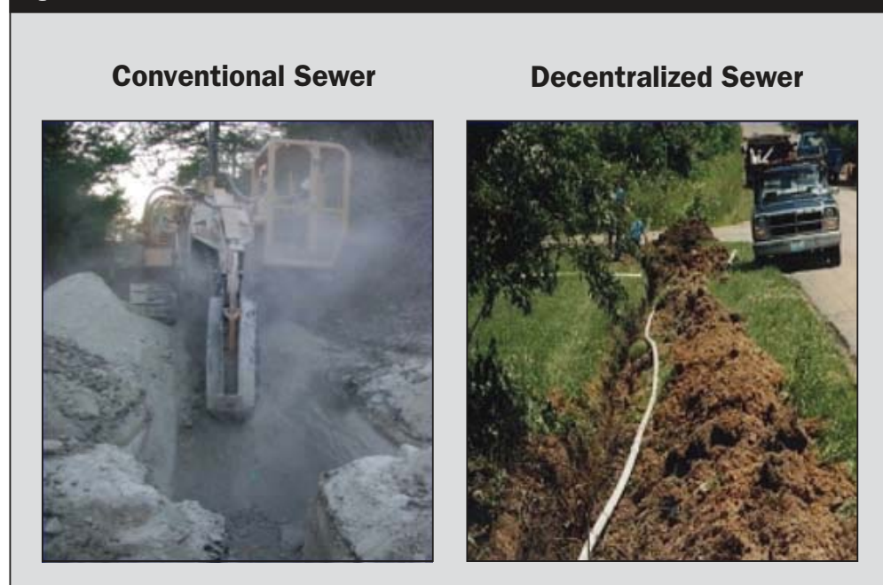
Figure 2. Conventional Versus Decentralized Collection Line Installation
